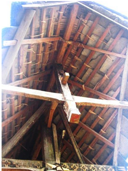
Figure 4. Stone as roof material on Tongkonan House (Source: Manurung, 2011)
