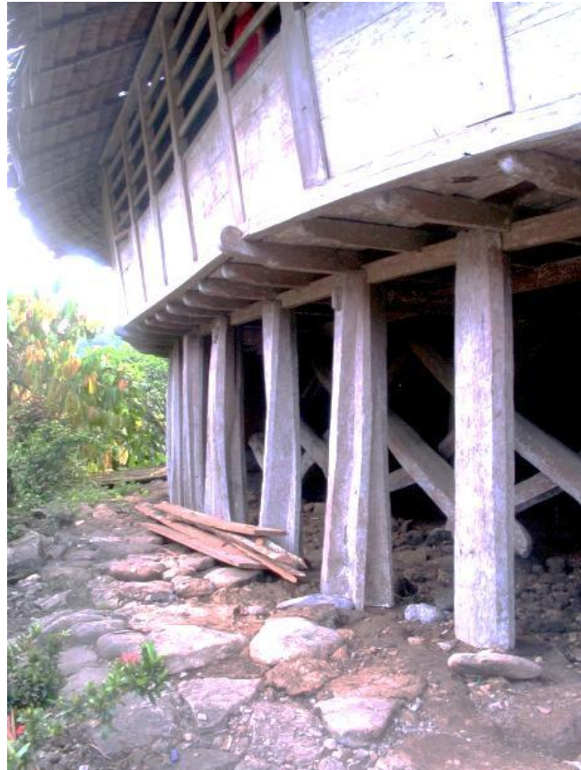
Figure 6. Stilt house is a problem solving for humidity. (Source: Author)
