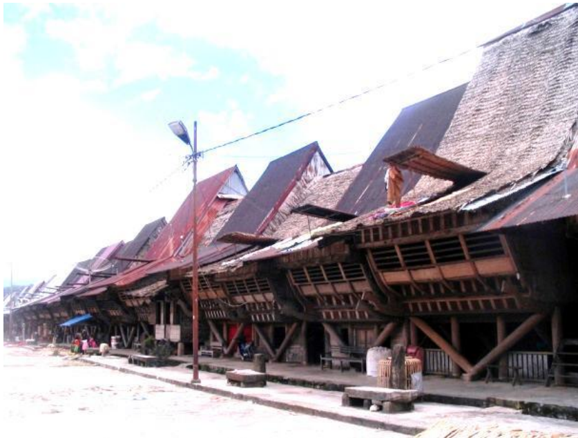
Figure 2. V-Shape structure system is a structural respond to lateral load caused by earthquake.
