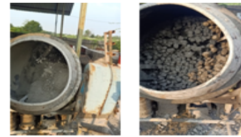
Gambar 2.2 Proses mixing beton umur 24 jam
