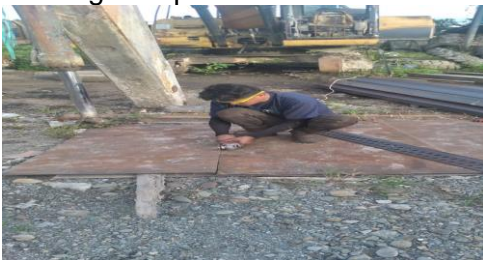
Gambar 2: Memotong besi plat
