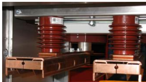
Gambar 4. Cable Compartment
