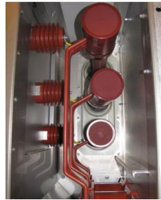
Gambar 2. Busbar Compartment
