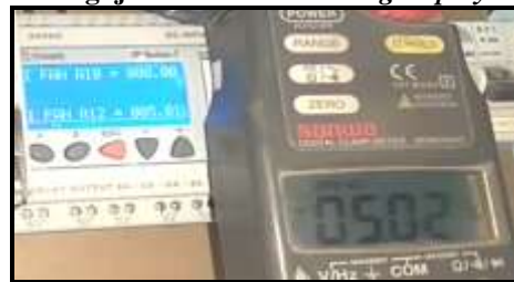
Gambar. 4.15 Pengujian sistem monitoring arus fan pendingin VSD.
