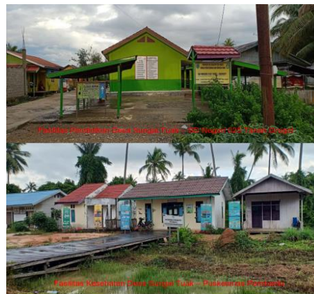
Figure 3. Facilities owned by Sungai Tuak Village
