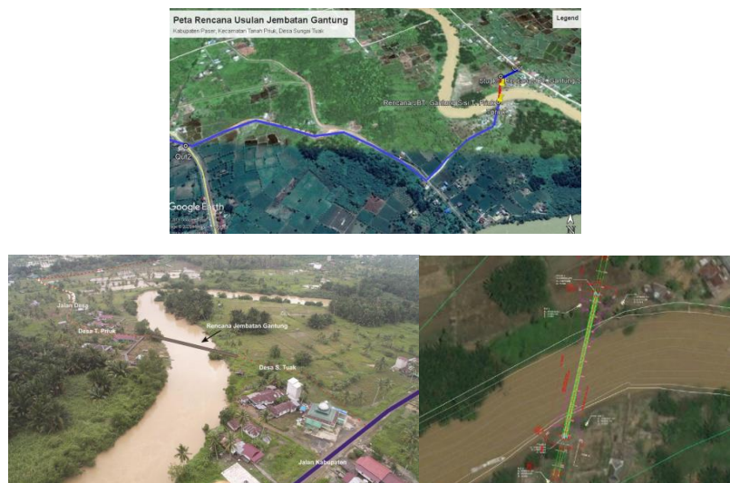
Figure 4. Field sketch of Tuak River Suspension Bridge site, Sungai Tuak Village
