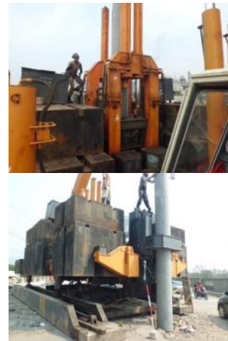
(a) Main Piling System (b) Side Piling Mechanism
