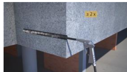
(a) Compressed air cleaning
