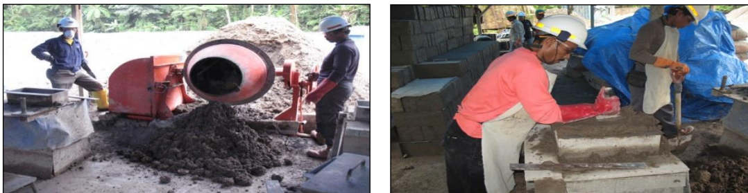
Fig. 3. Mixing and Compacting Process
