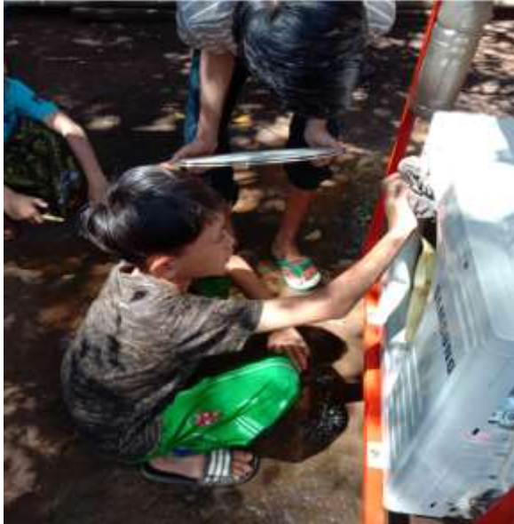
Gambar 5. Perawatan bagian outdoor AC
