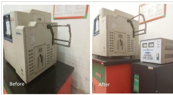
Fig. 7. Installation of silicon gel/stabilizer
