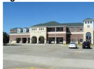
Gambar 1.: Orange Central Fire Station
