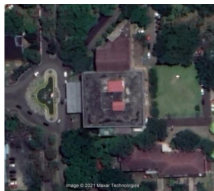
Figure 5 View of the Rectorate Building
