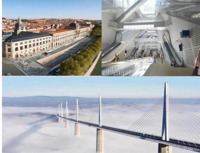
Fig. 10: Construction by Acciona
