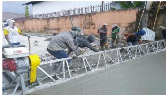
**Gambar 6. Vibratory Truss Screed**
