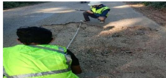
**Gambar 20.** Lubang (*Potholes*)
