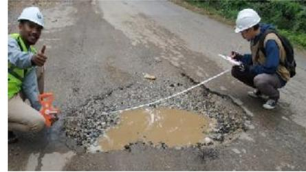
**Gambar 27.** Lubang (*Potholes*)
