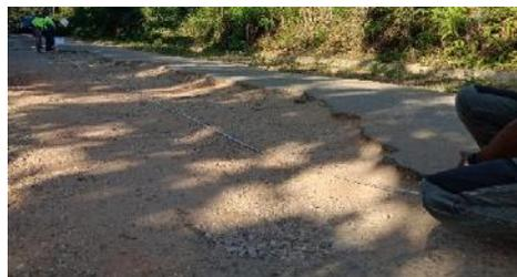
**Gambar 10.** Lubang (*Potholes*)
