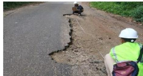
**Gambar 14.** Lubang (*Potholes*)
