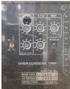
Figure 3 Setting Range Over-Current Trip
