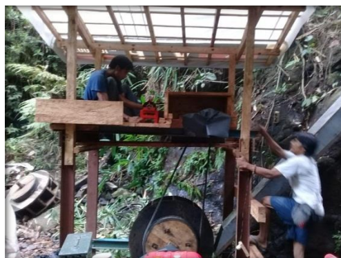
Gambar 13. Instalasi turbin-generator
