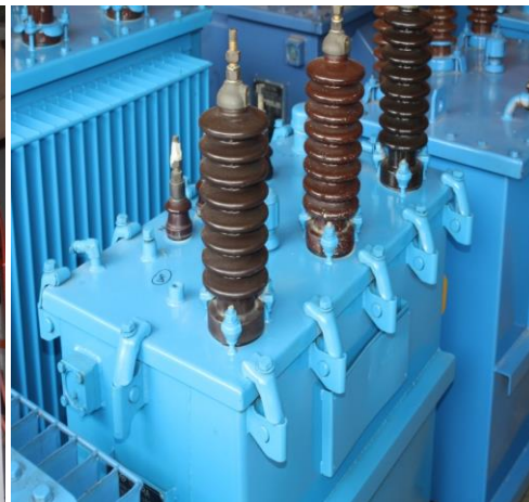
Gambar Bushing Transformator
