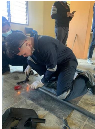
Figure 2. Sikap Kerja Proses Pengelasan
