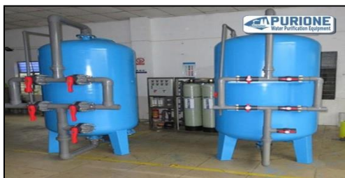
Figure 9. Carbon Filter (Source: PT. Nulab Pharmaceuntical Indonesia)
