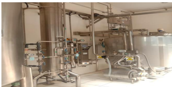
Figure 3. Mix Bed Water (Source: PT. Nulab Pharmaceutical Indonesia)
