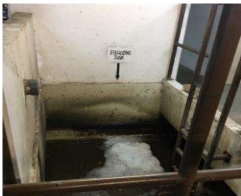
Gambar 8 Equalizing Tank
