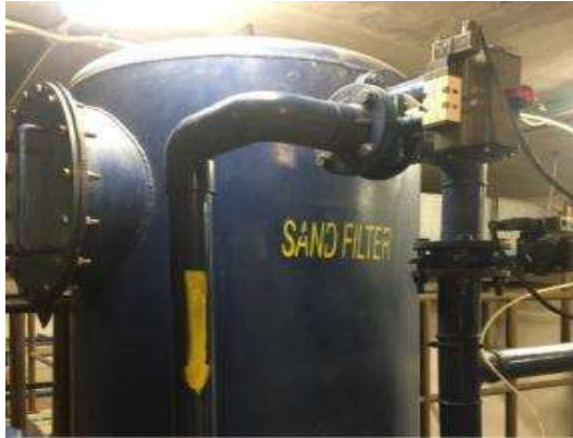
Gambar 18 Sand Filter
