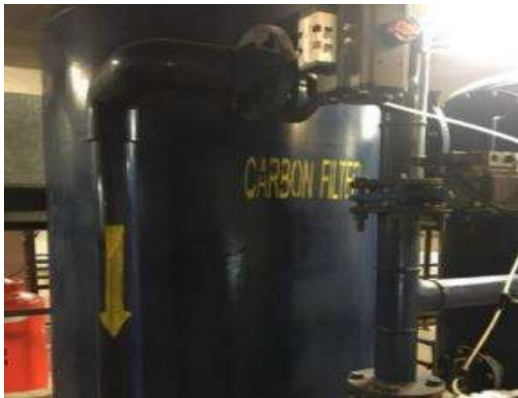
Gambar 19 Carbon Filter
