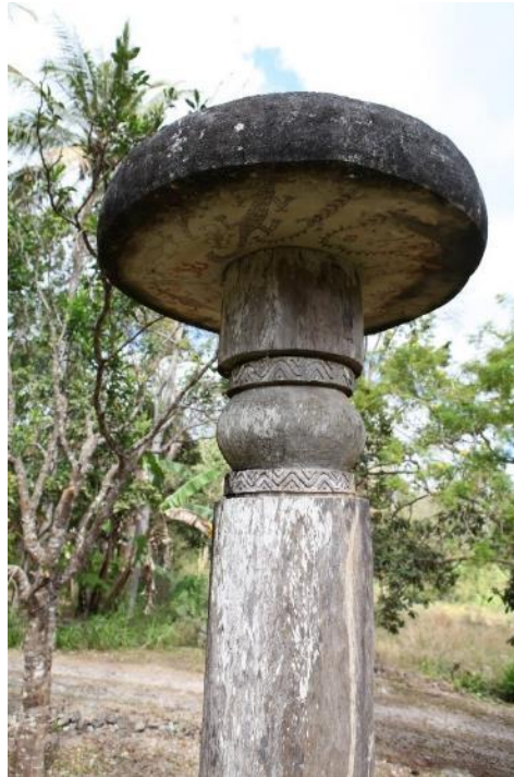
Fig. 3. Main pile (1 of four) of a ruinous Lopo in Nikiniki (near the rajas residence). The various different carvings and decorations can be seen very well.
