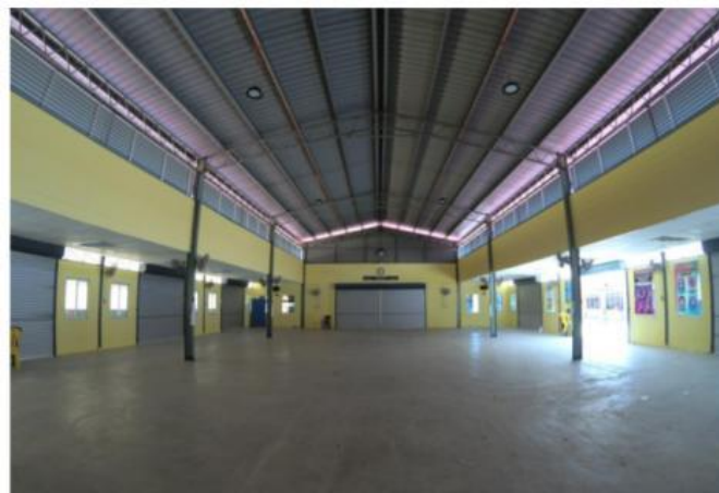
Fig. 8. Hall that used to accommodate flood victims.
