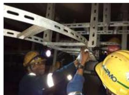
Gambar 6.3. Pemasangan HDG Carriage Bolt & din 980 Nut
