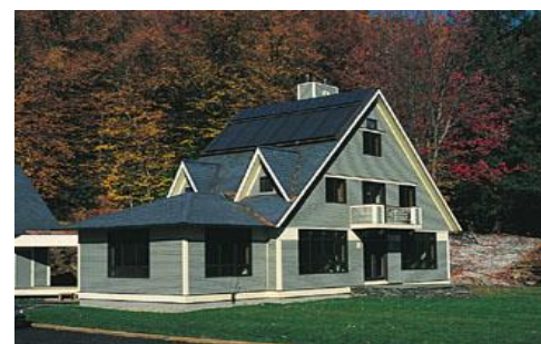
(b) Luxury home solar panel application
