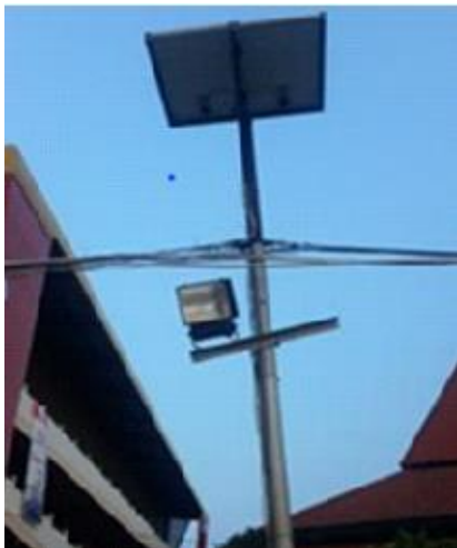
Gambar 10. Pemasangan panel surya 2x100WP
