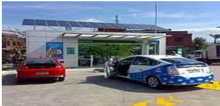
Fig. 6 Battery Charging Station in Rio de Janeiro, Brazil (Using Solar Energy)
