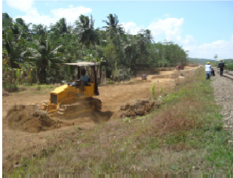
Gambar 1. Proses Pembersihan ( clearing )
