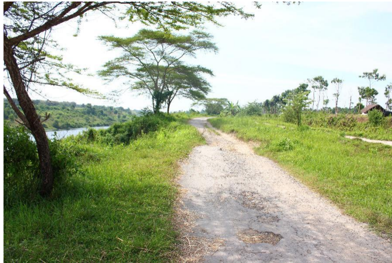
Figure 9. Inspection road of Plangwot Floodway in Lamongan, Indonesia
