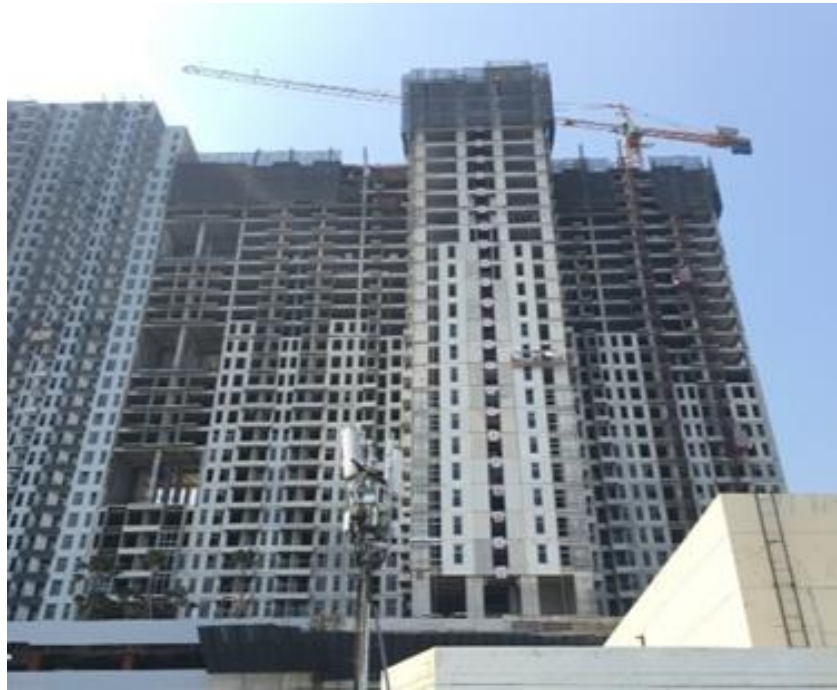
Fig.1 Existing Front View
