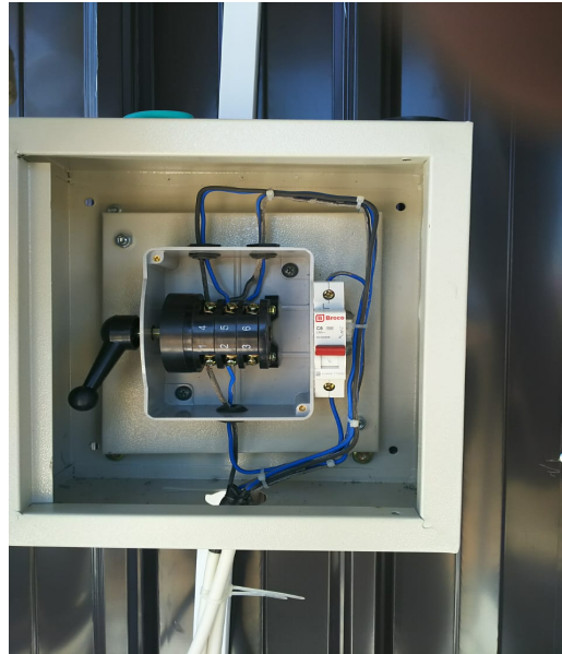
Gambar 8 Instalasi Box Panel
