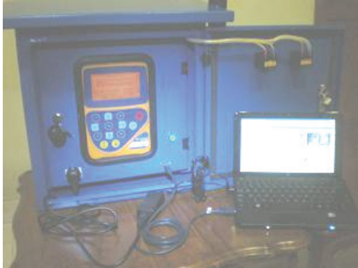
Gambar 21. Pengujian hardware dan software fixed monitoring system gas TPA
