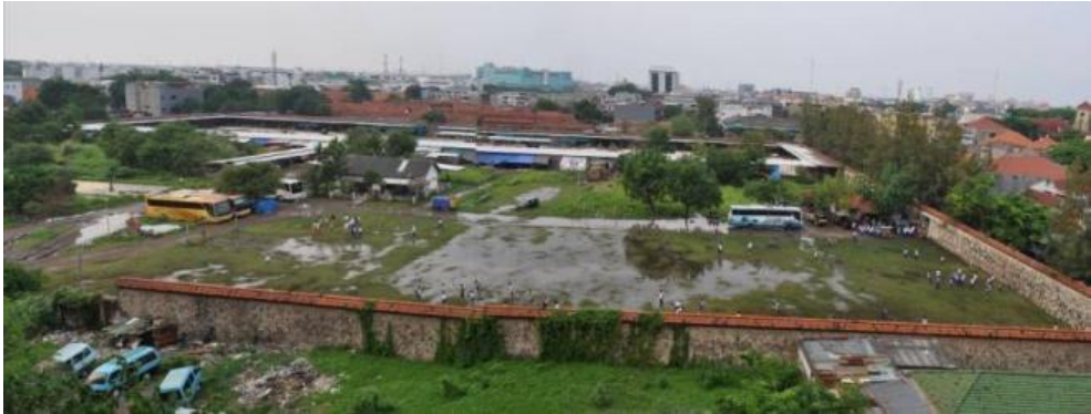
Figure 2. Koblen Prison View from BG Junction Parking Building at the South
