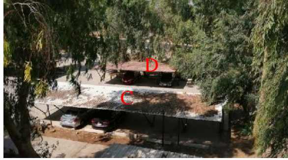
Figure 3. Cars garage sheds C and D.
