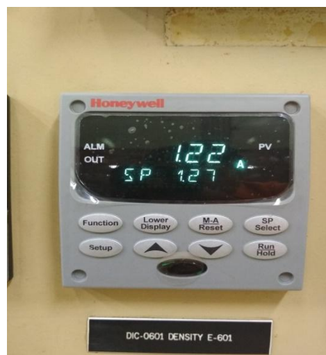
Gambar 4. Kontrol Panel densitas larutan Uranil Nitrat (UN) pekat
