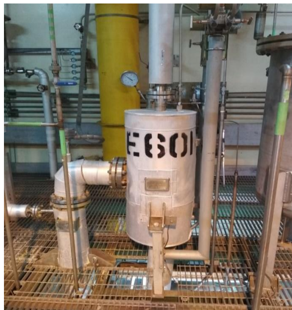
Gambar 1. Vertical Tube Evaporator
