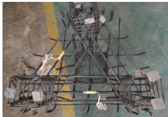
Gambar 3. Perakitan Baja Tulangan Metode Strut and Tie Model
