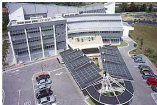
Figure 8: ZEO Building (Source: www.google.com)
