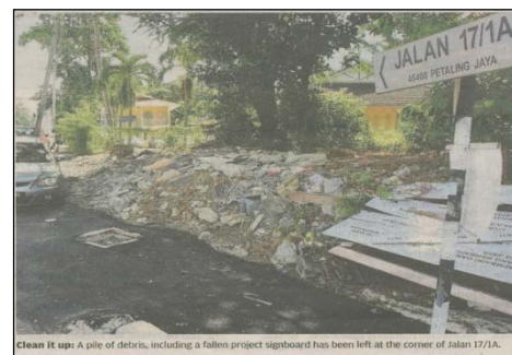
Figure 2: Construction debris along roadside [Source: The Star Newspaper 62]
