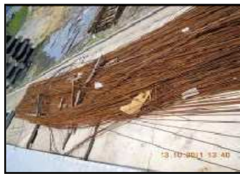
Figure 4. Surplus of reinforcement bar component waste
