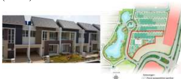
Figure 7: Houses at Cluster X, Perumahan Y, Gading Serpong, Tangerang Source: Private documentation, 2019
