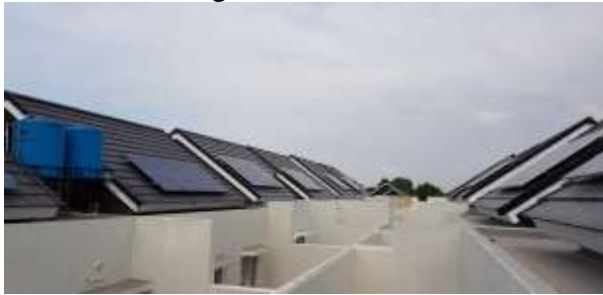
Figure 10: Solar Panel installation Source: Private documentation, 2019
