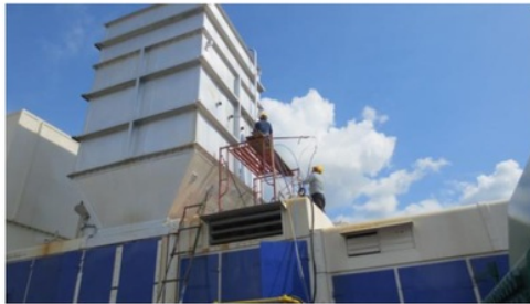
Figure 4 Installing Sampling Holes
