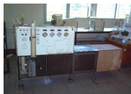
Gambar 3. Air cooled Chiller
