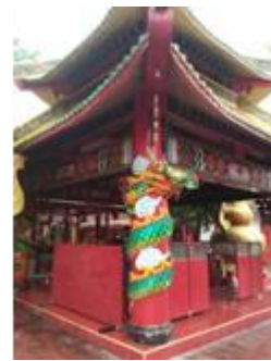
Gambar 11. Tampak gedung altar Thian Kong
