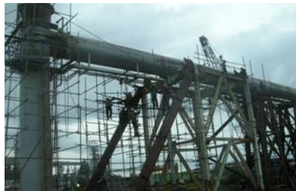
Gambar 6. Cara Penarikan Pipa Transfer Line
