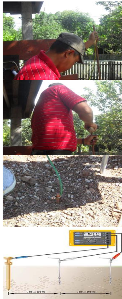
Gambar 4. Pemasangan Pembumian (Grounding) Single Point Ground
