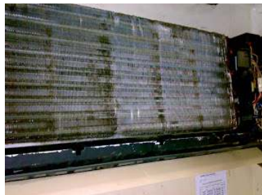
Gambar 2.3 Evaporator
