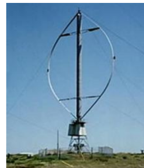
Gambar 3 Turbin Darrieus
