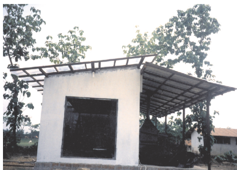
A. Bangunan pengeringan dengan radiasi panas matahari melalui atap ( Drying building with solar radiation passing through the roof )
