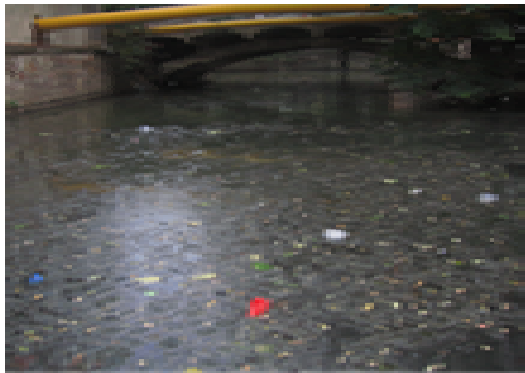
(c) Kondisi di Jembatan Xishan New Village
