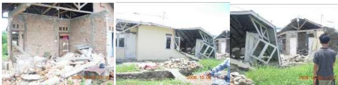
Figure 1. Condition of Masonry Houses after earthquake
